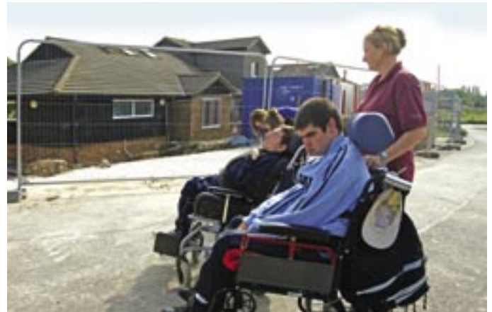
Residents and staff watch the building progress at Frances House
