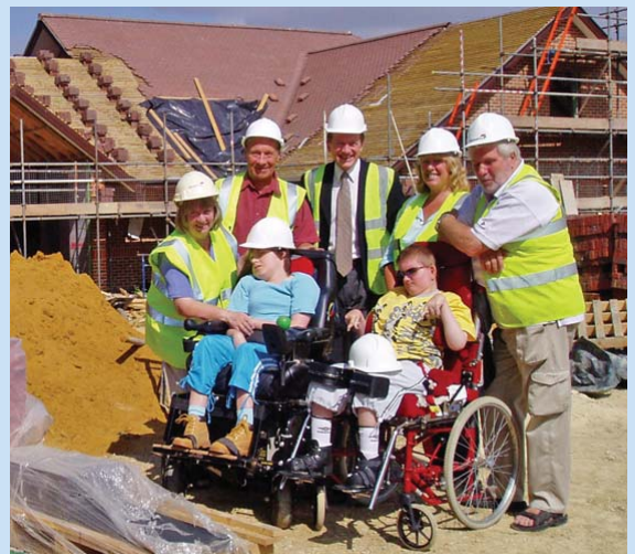
Graham Simmons (centre), pictured with visitors inspecting progress at Agape House, Hastings.
